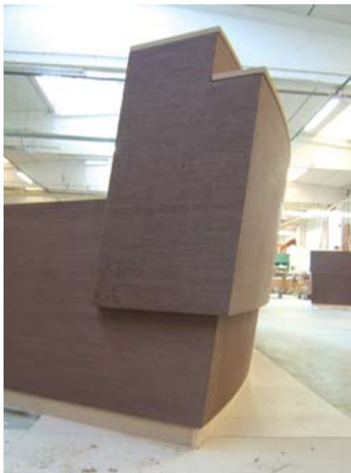
Reception in costruzione / Reception desk under construction
