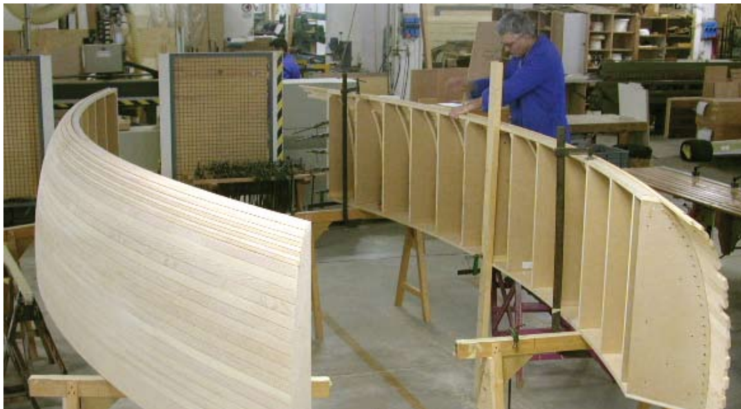
La “carena” in costruzione / “Boat keel” under construction
