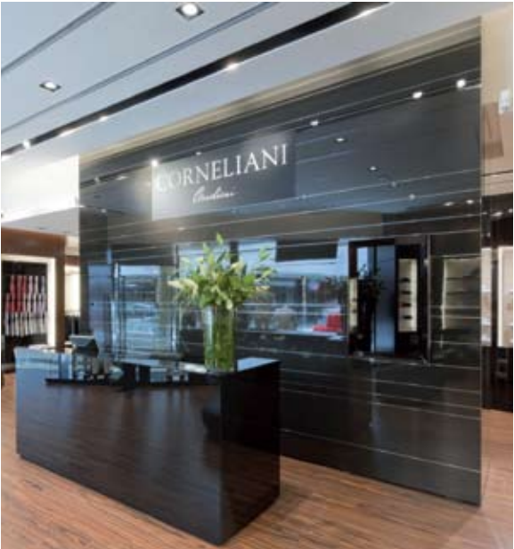
Banco cassa e parete retrocassa in carbonio con inserti in acciaio inox / Cash desk and rear wall in carbon fiber with stainless steel insets
